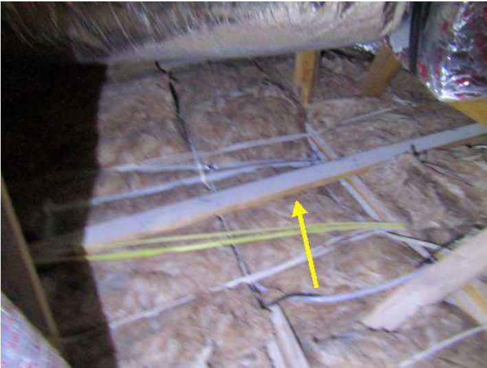
supply lines missing insulation, installation of pipe insulation is recommended.
