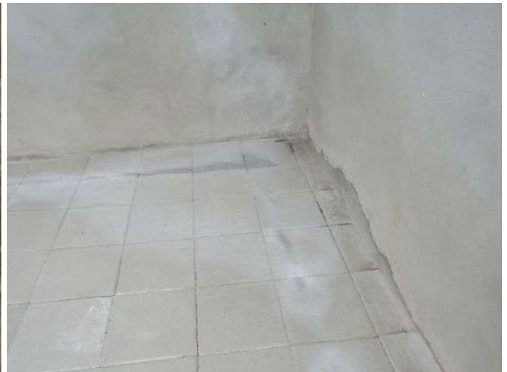
Visible erosion, recommendation of gutter installation throughout the house recommended.
