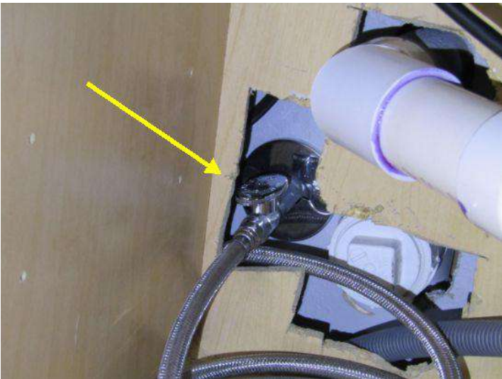
service valves are too far for servicing
