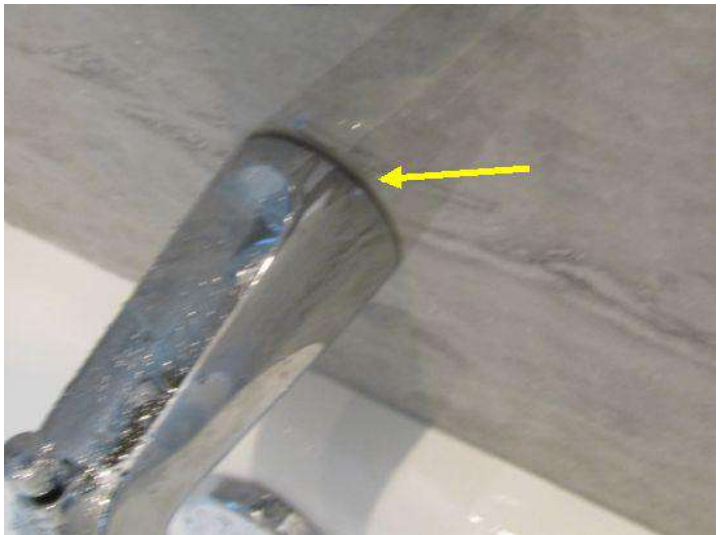
missing sealant at spout
