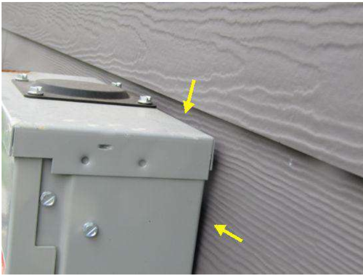
missing sealant
