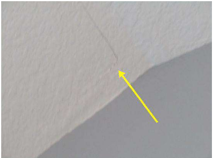
Small cracks on ceiling
