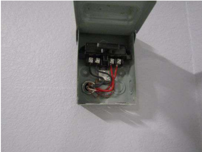
disconnect box missing interior cove.
