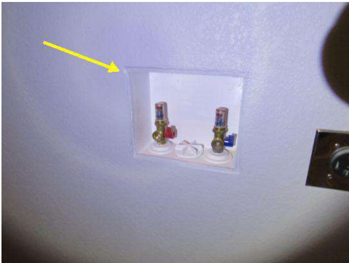
valve box missing cover
