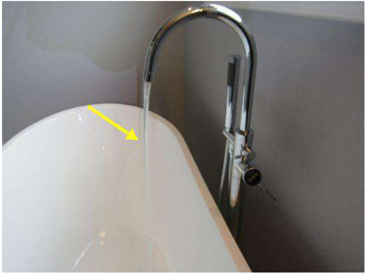
low water flow when cold water is turned on
