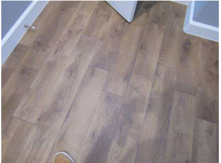
floor is warped in some areas repair is recommend before closing
