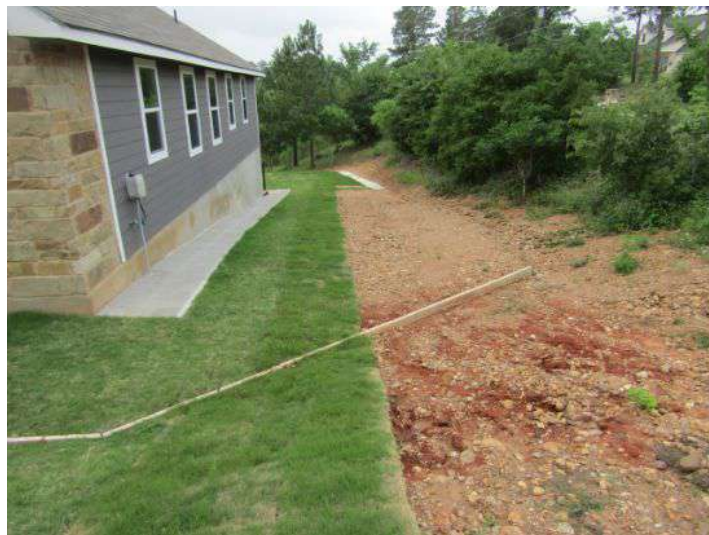
Visible erosion, recommendation of gutter installation throughout the house recommended.
